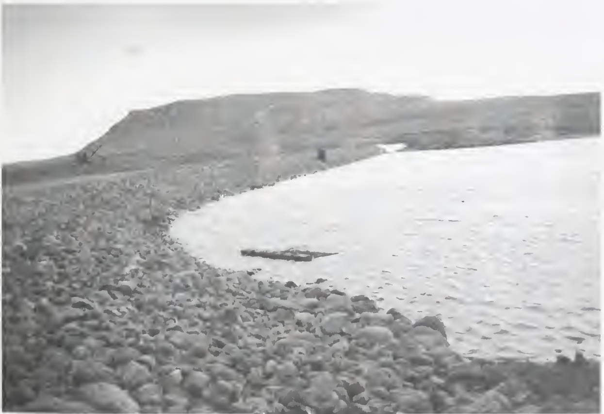
Browns Dam completed in 1934, Square Butte in the background
